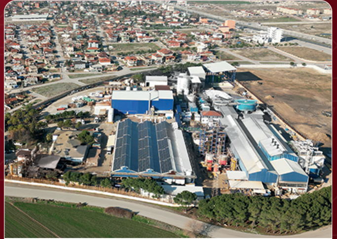
DENİZLİ Production Facility
